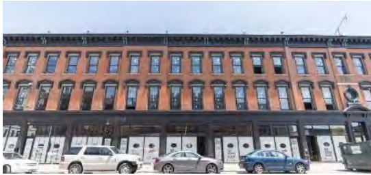
Boone Block, built in 2016, 9 homes
