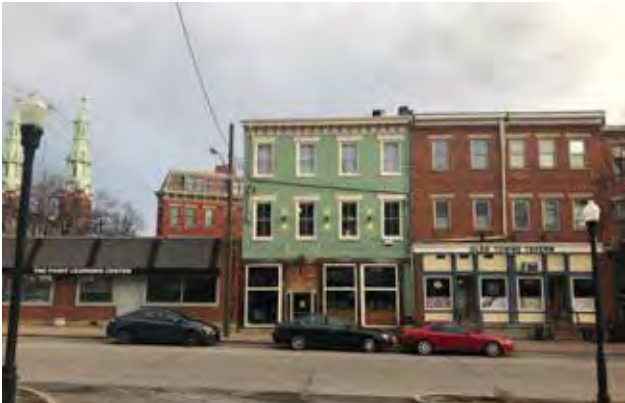
Figure 4.30. Example of existing stacked flats
