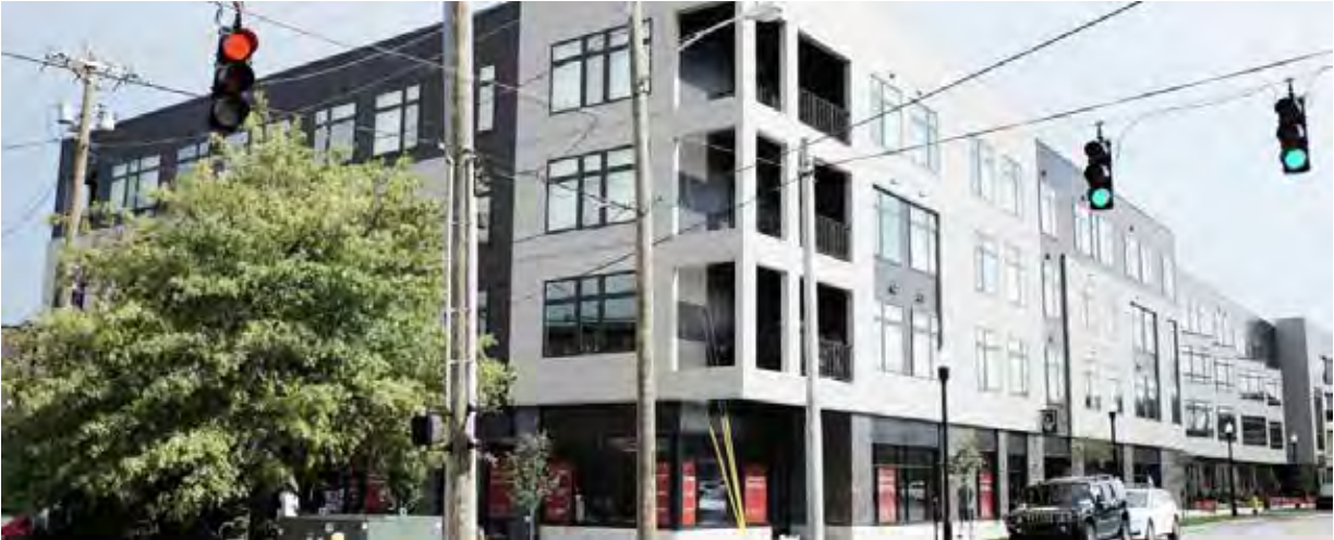
Figure 4.31. Example of existing multifamily residential
