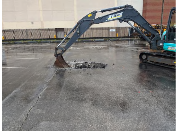
Photograph 6: Anomaly located in Survey Area #3 (auto repair northeast).
