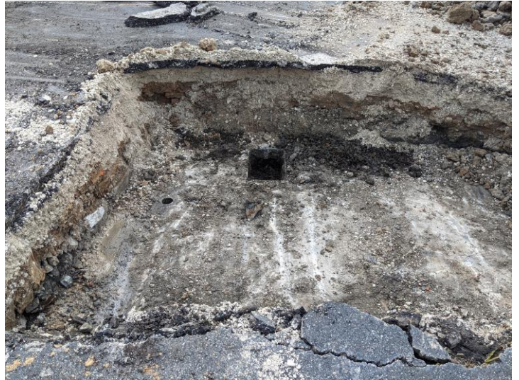
Photograph 2: View of the concrete vault excavated in Survey Area #7.
