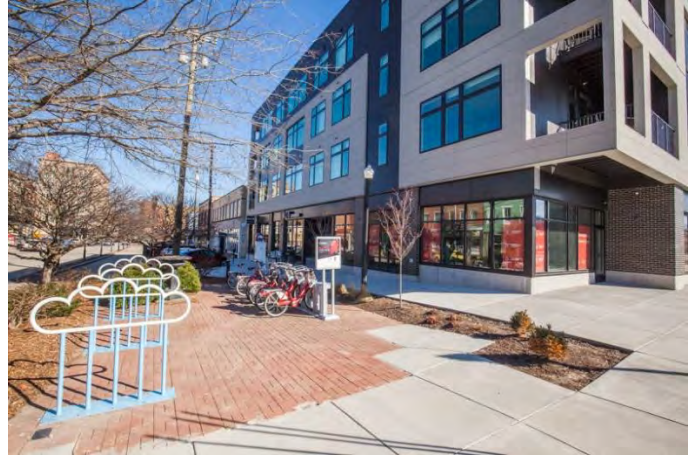
Example infill construction on West 7 th Street that implemented new storefronts and used similar proportions, heights, and rhythm of openings in other buildings found within the neighborhood
