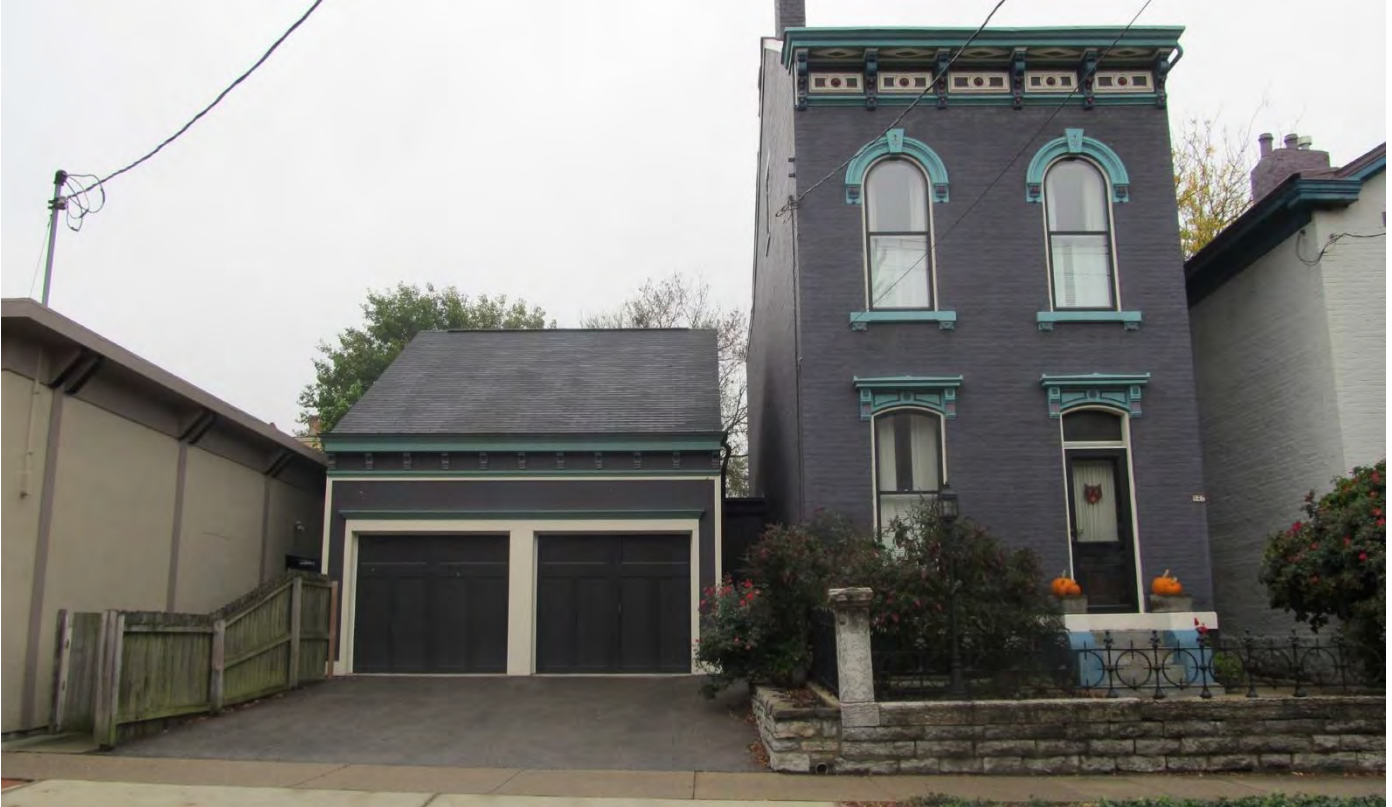
Example of appropriate new construction garage that is context sensitive and complimentary to the main building.
