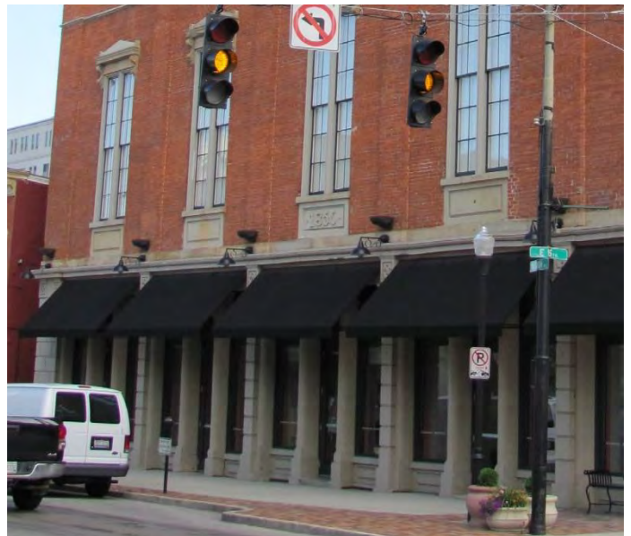
Example of awning broken up over a large span as to not obscure architectural elements
