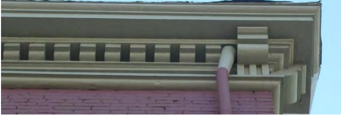
Appropriately painted box gutter and downspout system
