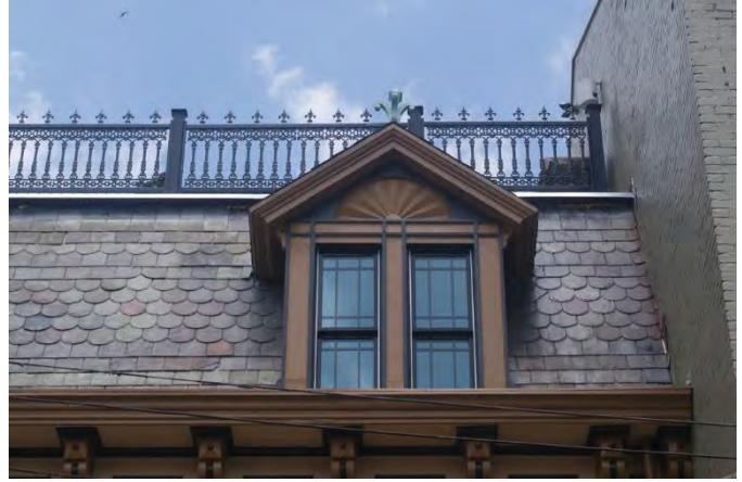
Metal roof cresting that was replicated to replace a missing element
