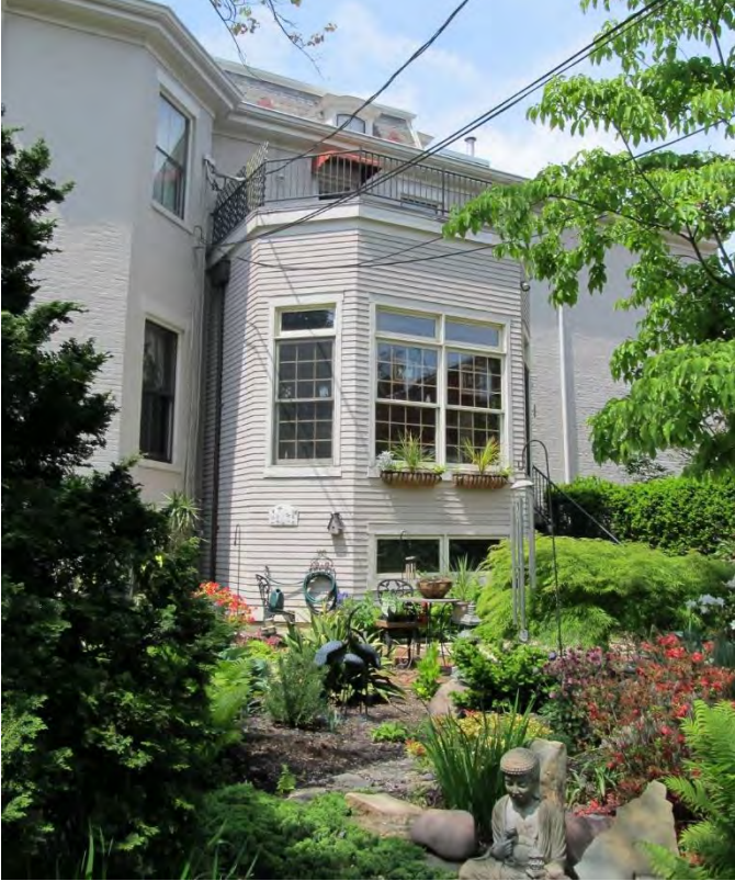
Example of an addition
