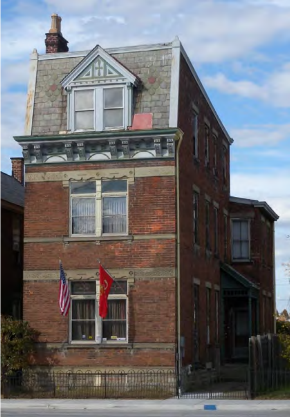
Example of underground utilities
