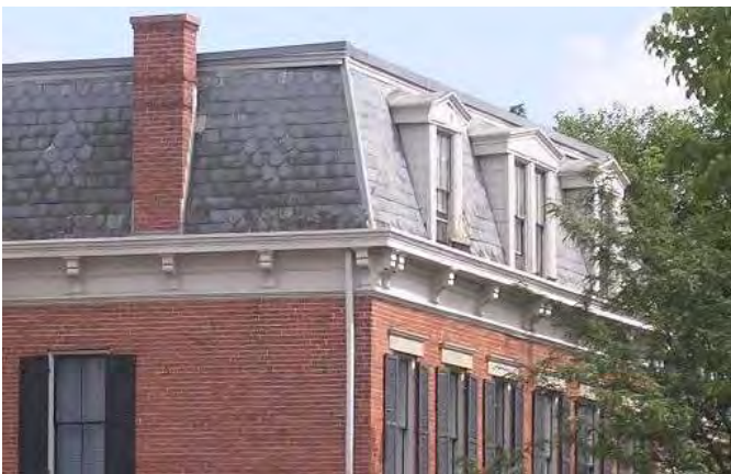
Mansard roof with original slate shingle roof and dormers
