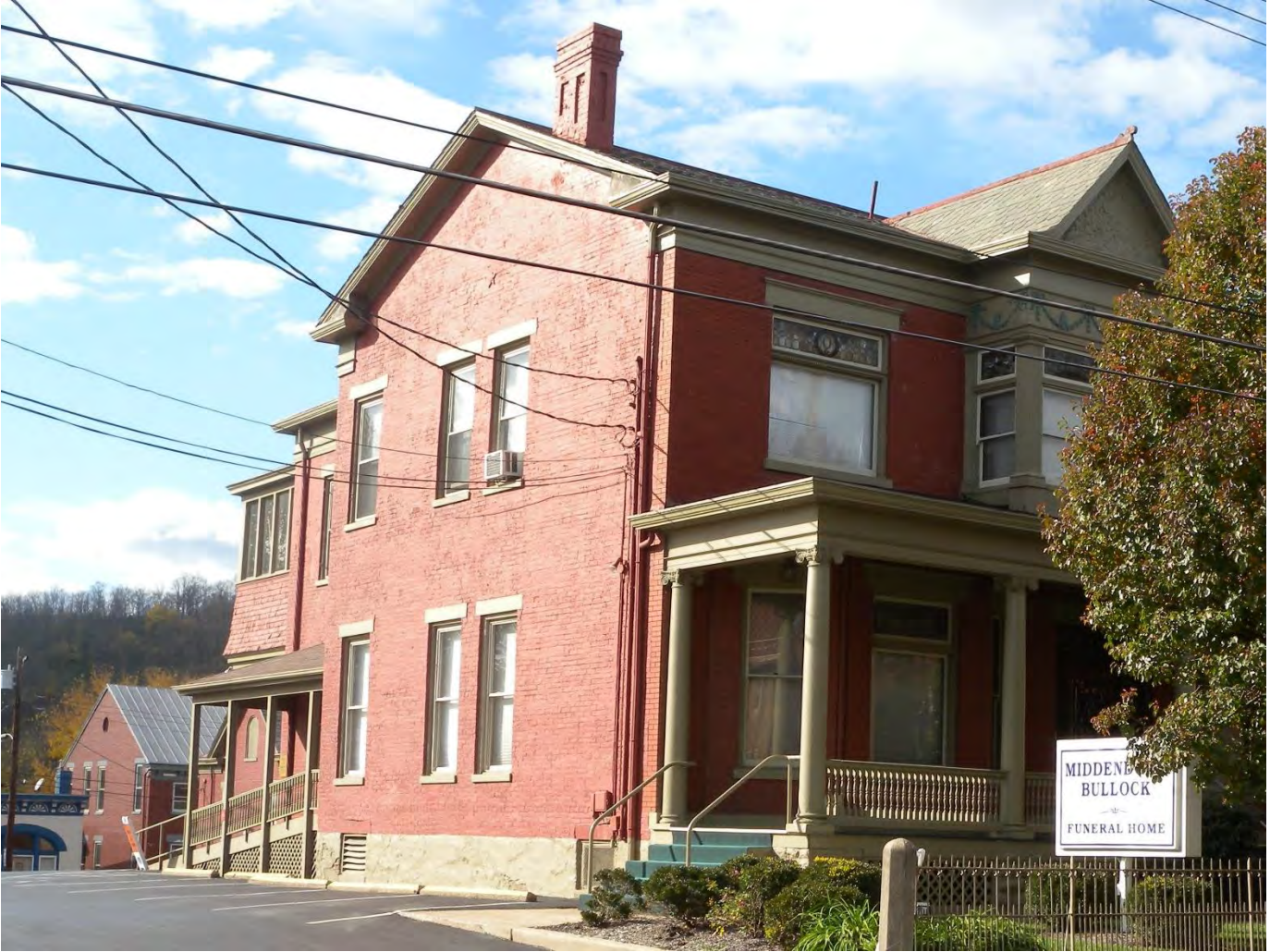
Example of accessibility ramp on the rear of a building
