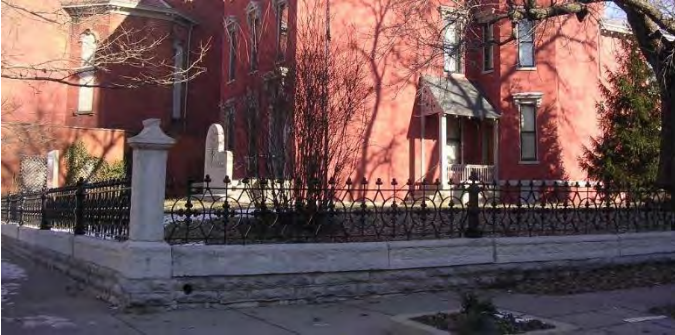
Example of stone retaining wall with iron fence
