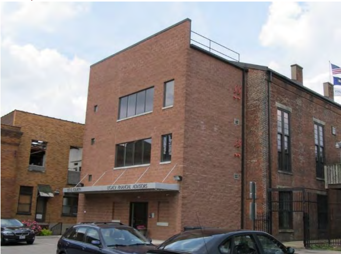
Example of an addition
