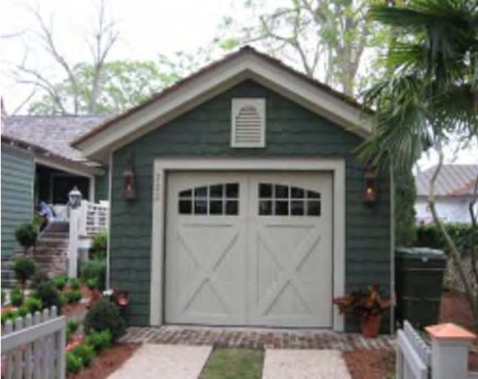
Appropriate new construction single-car detached garage
