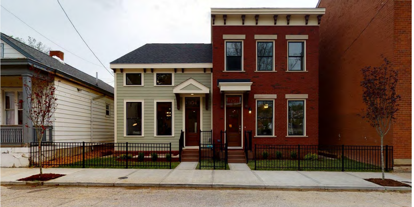
New construction on a formerly unimproved lot in MainStrasse
