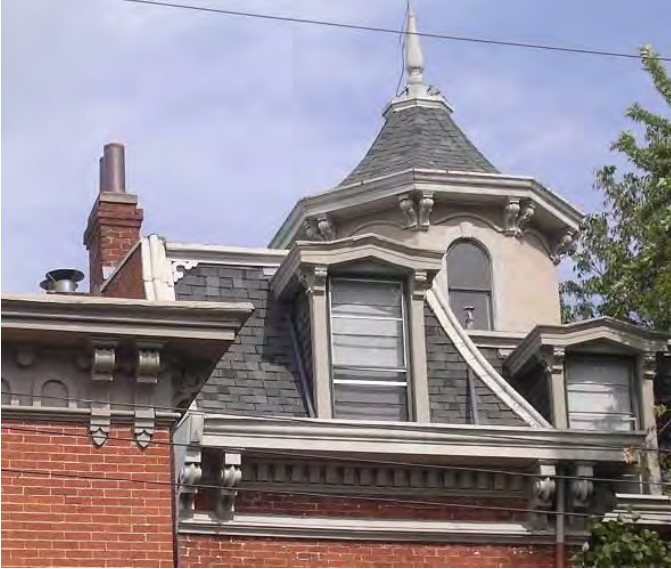
Examples of dormers, chimney, cornice, and eaves
