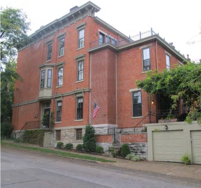
Example of an elevator addition on the side of a building
