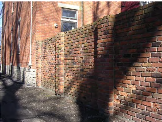
Example of brick privacy wall
