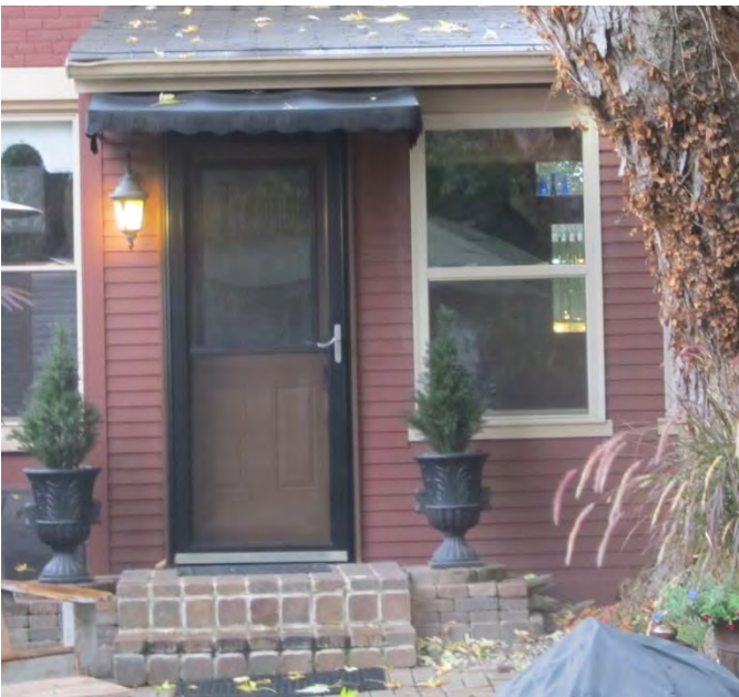
Example of rear entrance on a residential structure
