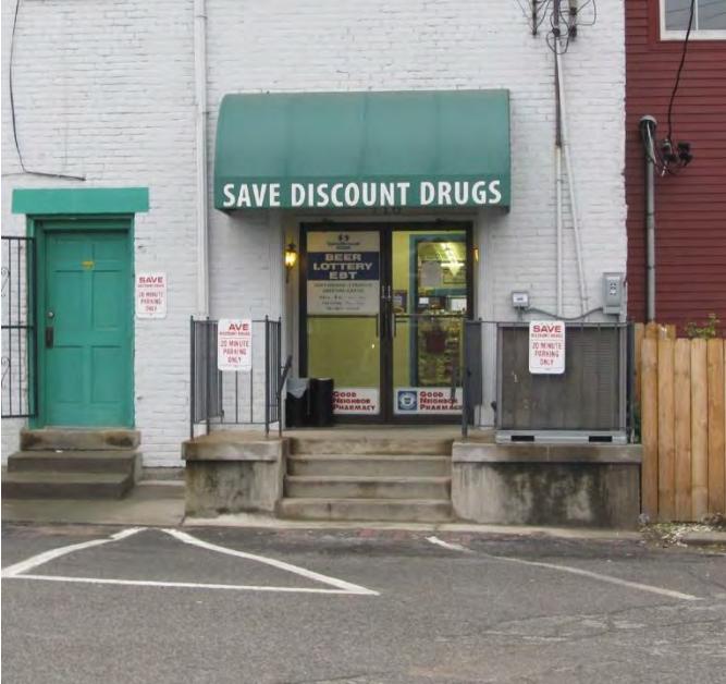
Example of rear entrance on a commercial building
