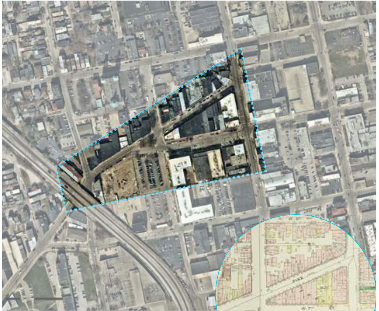
ABOVE: DUVENECK SQUARE DISTRICT OUTLINE RIGHT: 1886 SANBORN MAP OF PUBLIC MARKET HOUSE ON 7TH STREET
