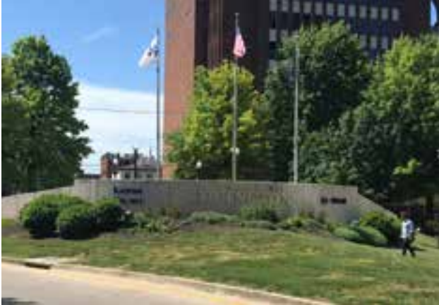
Current Gateway Wall Sign- The current sign wall located at the terminus of the Roebling Bridge limits views into and out of the district.
