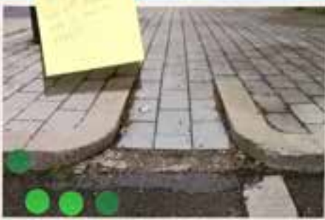
1 PEDESTRIAN ACCESSIBILITY Existing curb and ramp configuration limits flexibility and does not meet current ADA standards
